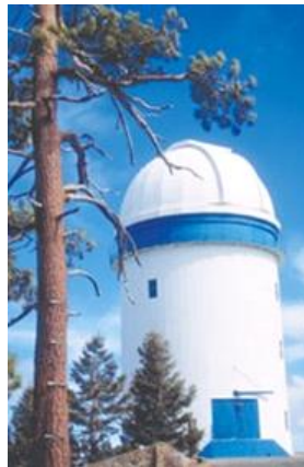
Figure 4.1 An image of the San Pedro Martir facilities in Ensenada Mexico 18
